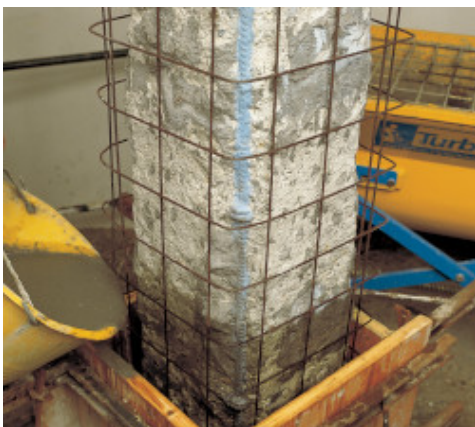
Pouring into a formwork
