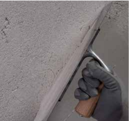
Smooth texture skimming mortar on existing render.
