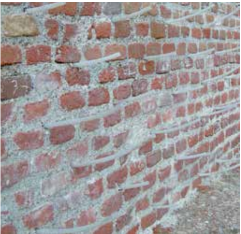
Consolidation of a brick parapet wall.
