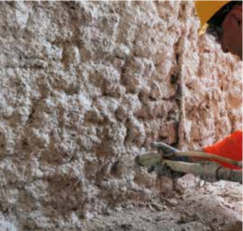
Application by rendering machine on stone masonry.
