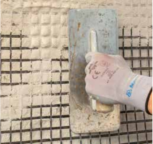
Application of mesh for FRCM strengthening reinforcement.
