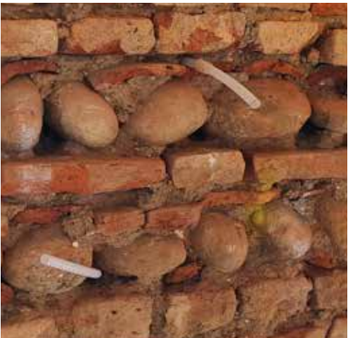
Consolidation of “rubble masonry” stone masonry.
