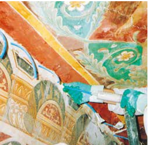
Injection of Mape-Antique F21 to consolidate the adhesion of decorated render.
