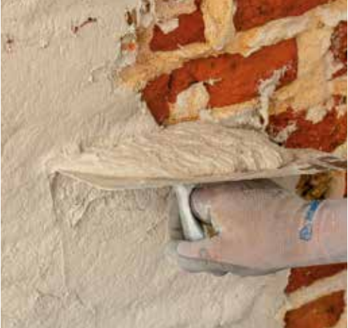
Application by trowel on brick masonry.
