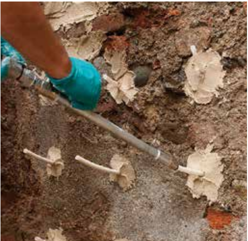
Injecting with low-pressure pump.
