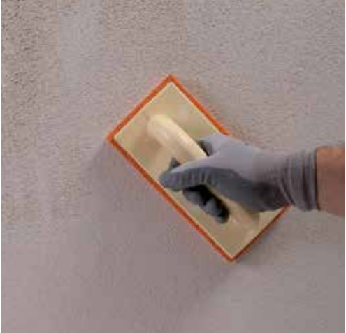
Finishing off Mape-Antique NHL ECO Rasante Grosso with a sponge float.
