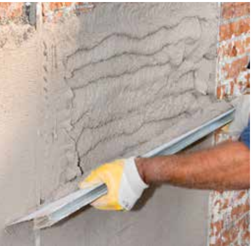
Compacting the transpirant render with a straightedge.
