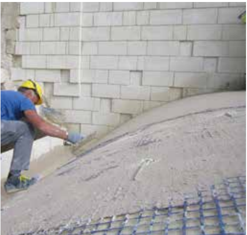
Extradossal reinforcement of tuff vaults (CRM).
