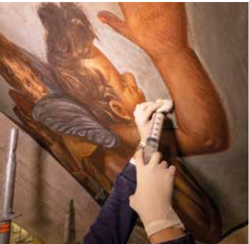
Injection of Mape-Antique F21 to re-establish the adhesion of decorated render.
