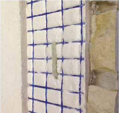
“Reinforced” plaster with glass fibre mesh (CRM).
