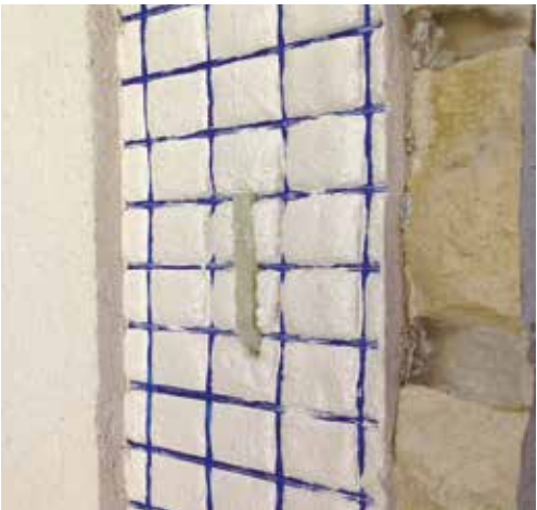
Plaster “reinforced” with glass fibre mesh (CRM).
