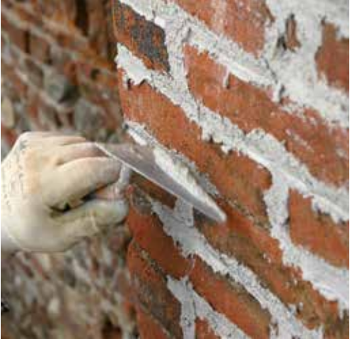
Pointing brick masonry.
