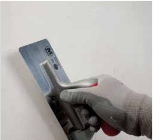
Application of the second layer of Mape-Antique FC Ultrafine .
