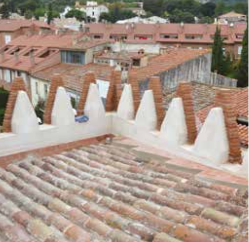
Red brick pinnacle reinforcement castings.
