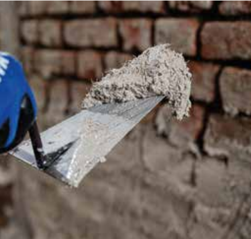
Application by trowel on brick masonry.
