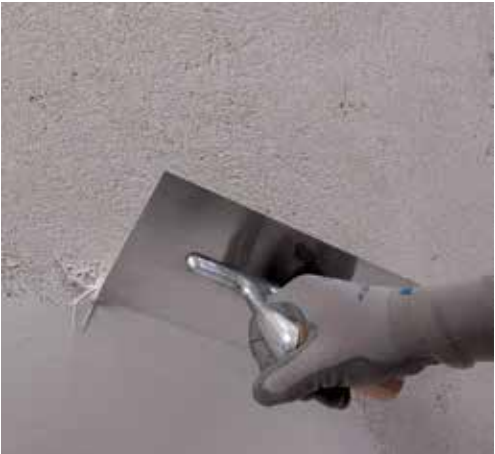
Application of the first layer of Mape-Antique FC Ultrafine .
