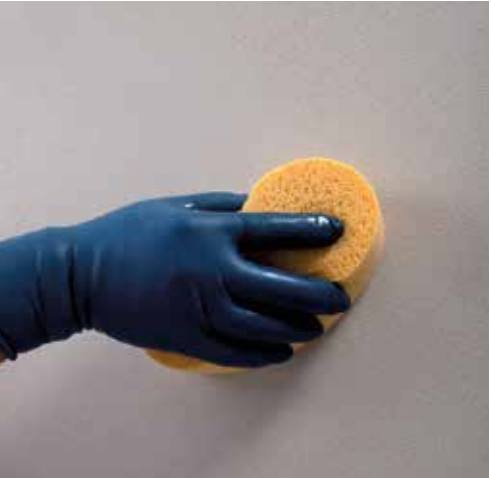
Finishing off Mape-Antique NHL ECO Rasante Civile with a sponge float.
