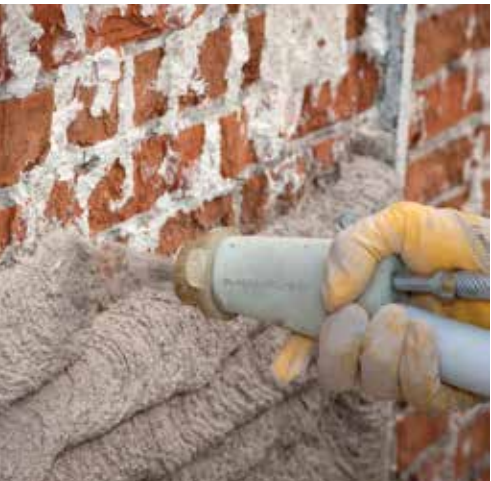
Application by trowel on brick masonry.
