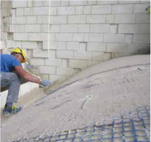
Extradossal reinforcement of tuff vaults.
