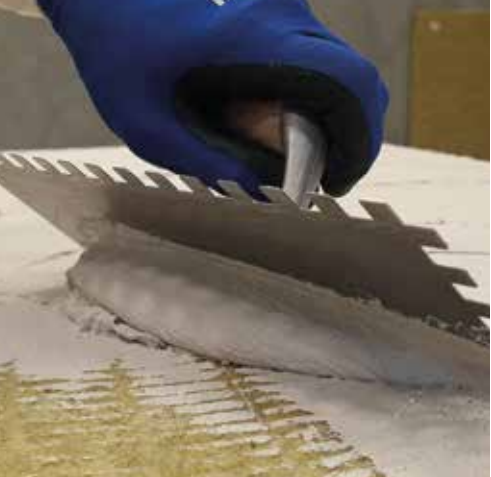
Application as adhesive on panels rock wool panels.
