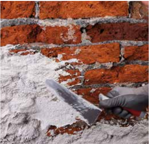
Application by trowel on brick masonry.
