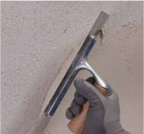
Coarse texture skimming mortar on existing render.
