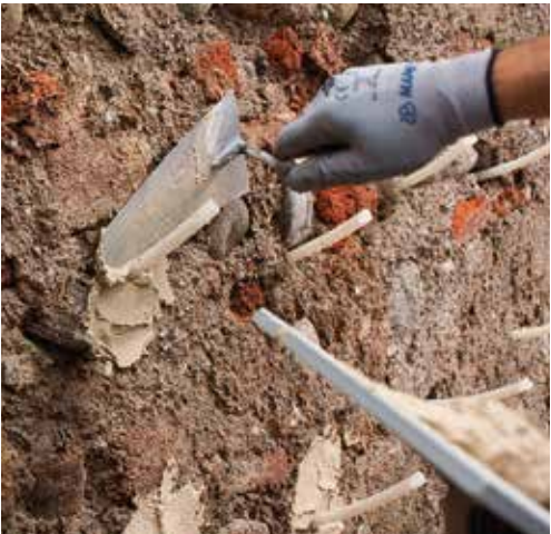
Fastening the small rubber injection tubes in place with Mape-Antique Allettamento .
