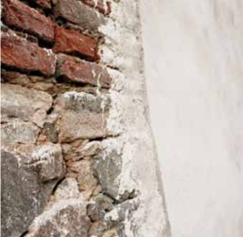
Application as render on mixed masonry.
