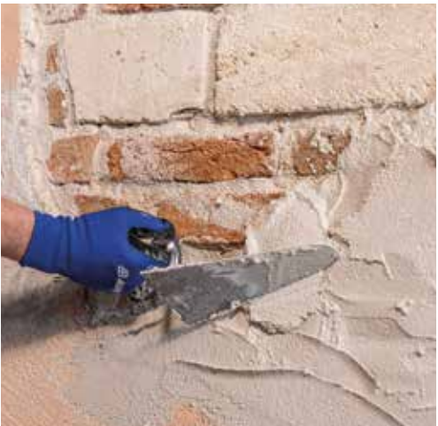
Rebuilding an existing render.
