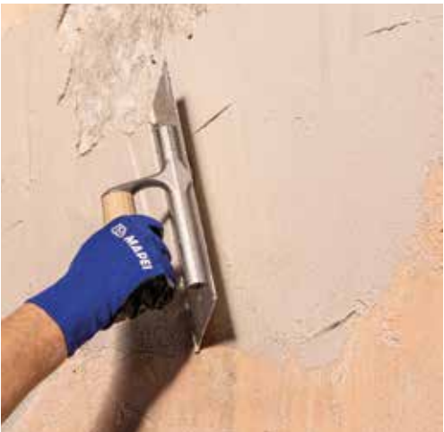
Levelling off an existing skimming coat.
