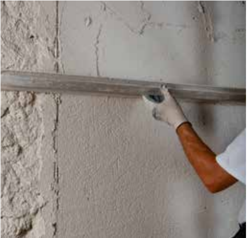
Compacting the dehumidifying render with a straightedge.
