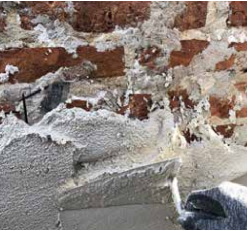
Application by trowel of single-layer dehumidifying plaster on brick masonry.
