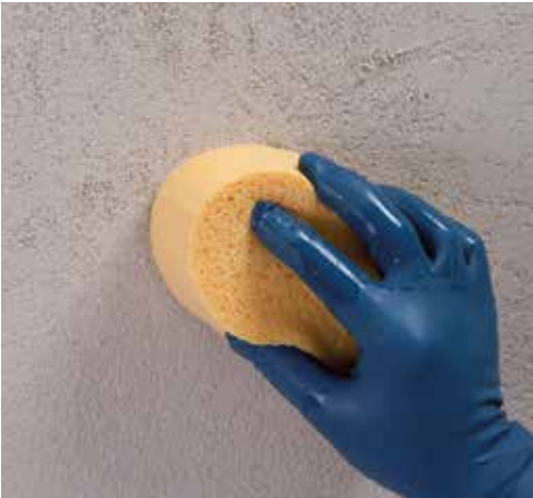
Finishing off Mape-Antique FC Grosso with a sponge float.
