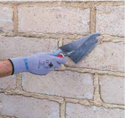
Pointing tuff masonry.
