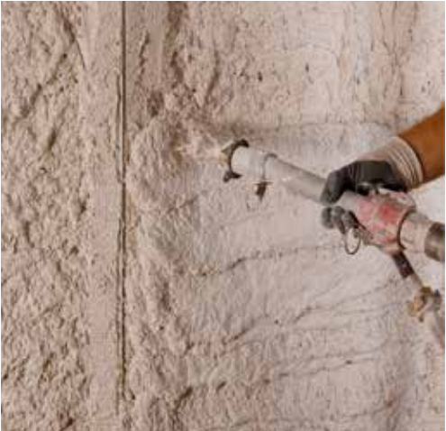
Application by trowel on brick masonry.
