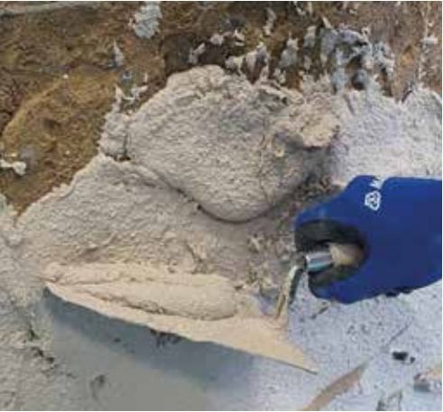
Application by trowel of single-layer dehumidifying plaster on tuff masonry.
