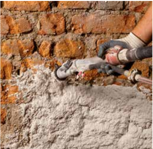
Application with rendering machine.
