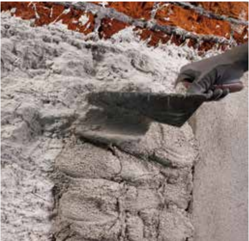
Application by trowel on brick masonry.
