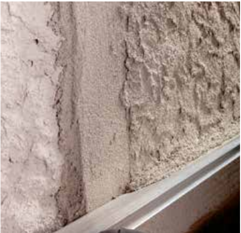
Compacting the dehumidifying render with a straightedge.
