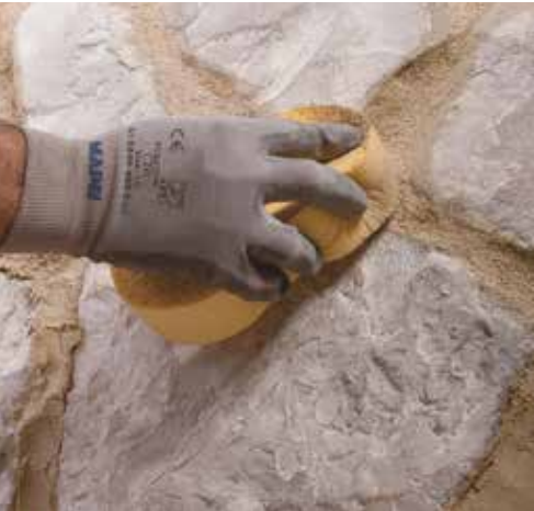
Finishing off Mape-Antique Allettamento with sponge.
